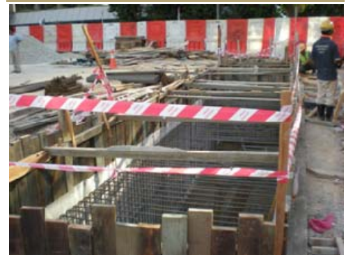
Figure 5: Some underground works have also commenced
