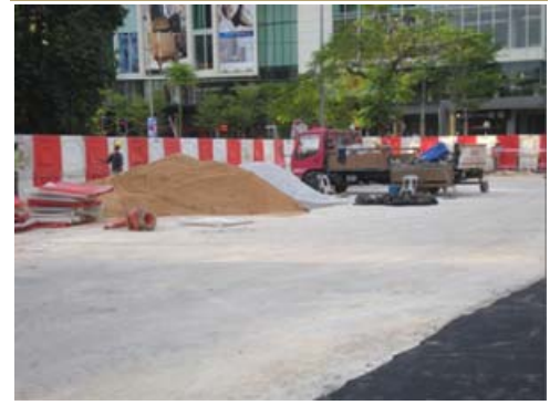
Figure 3: Site clearing for the LRT line to pass through has begun
