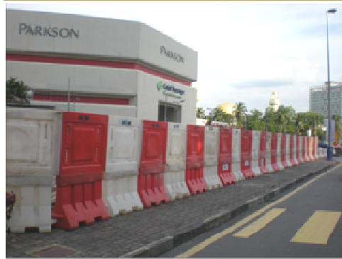
Figure 2: LRT site in front of Subang Parade is now barricaded
