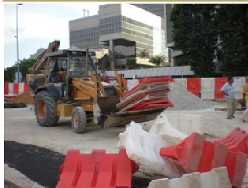
Figure 4: Tractors being mobilized at the LRT site
