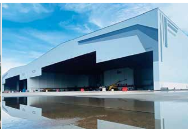
The Refurbishment of Main Building and Infrastructure Works at Subang Engineering Complex A, Sultan Abdul Aziz Shah Airport (SECA)
