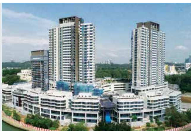
Ongoing Project of the Putrajaya Mixed Development Project (8MD3)
