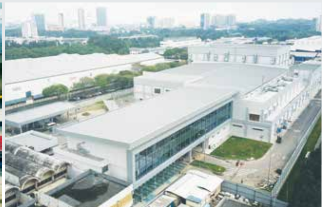
Completed Phase 2 of the MINT Modernisation Project at Shah Alam for Bank Negara Malaysia
