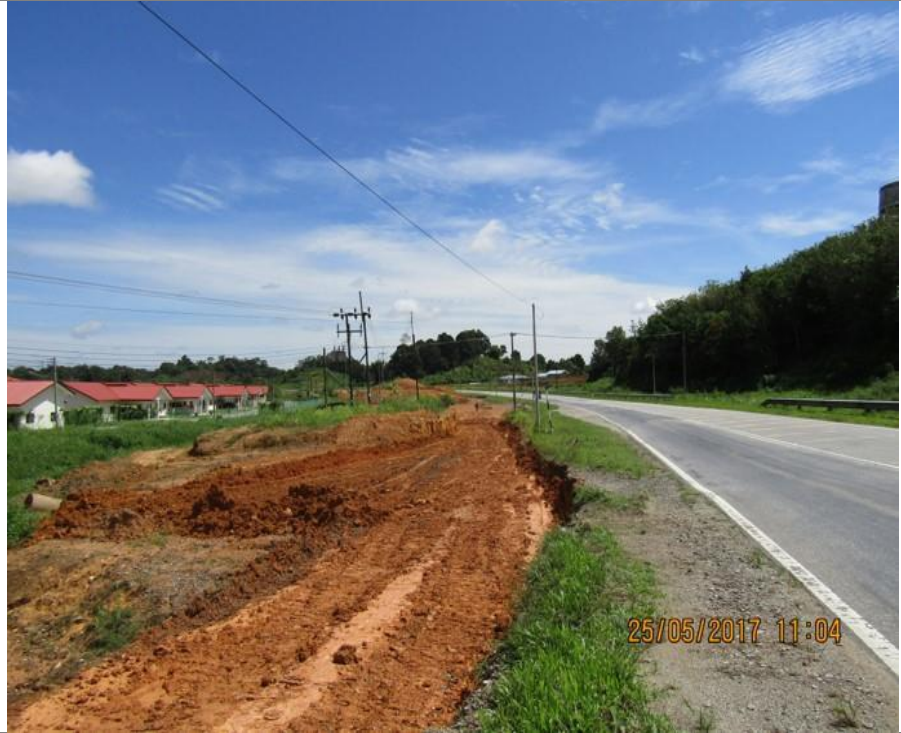
Chart 9 : Pan Borneo Works Package 5: Embankment fill in progress (Betong Section)
