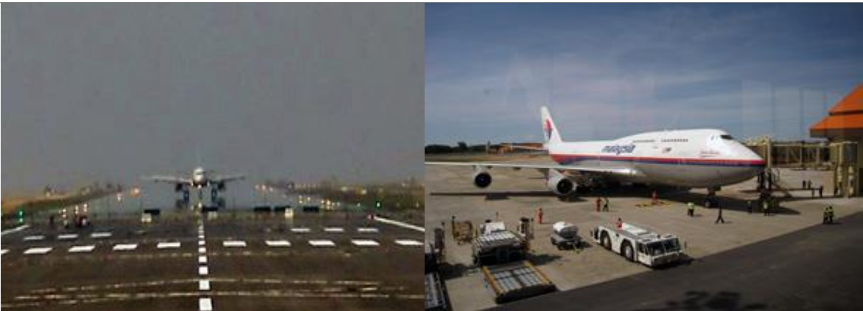
Chart 16 : Kuala Terengganu Airport runway extension (Package 3)
