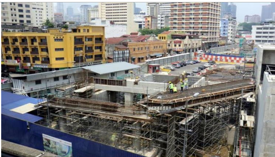
Chart 4 : Construction works for the MRT 1 Pasar Seni (Central Market) Underground Station
