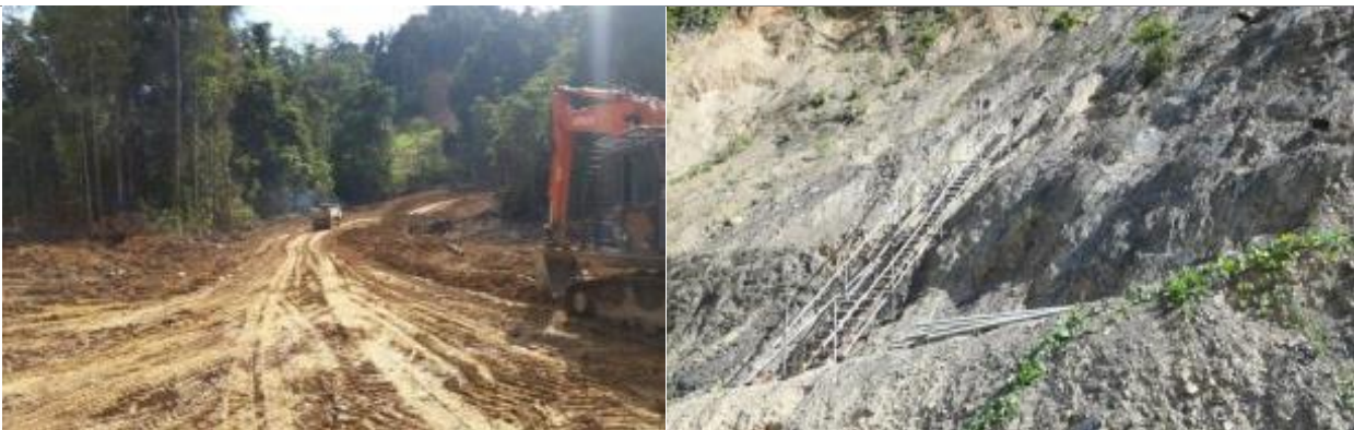
Chart 11 : Sabah Sarawak Gas Pipeline - repair & maintenance of access roads, slope stabilization works (Sarawak section)
