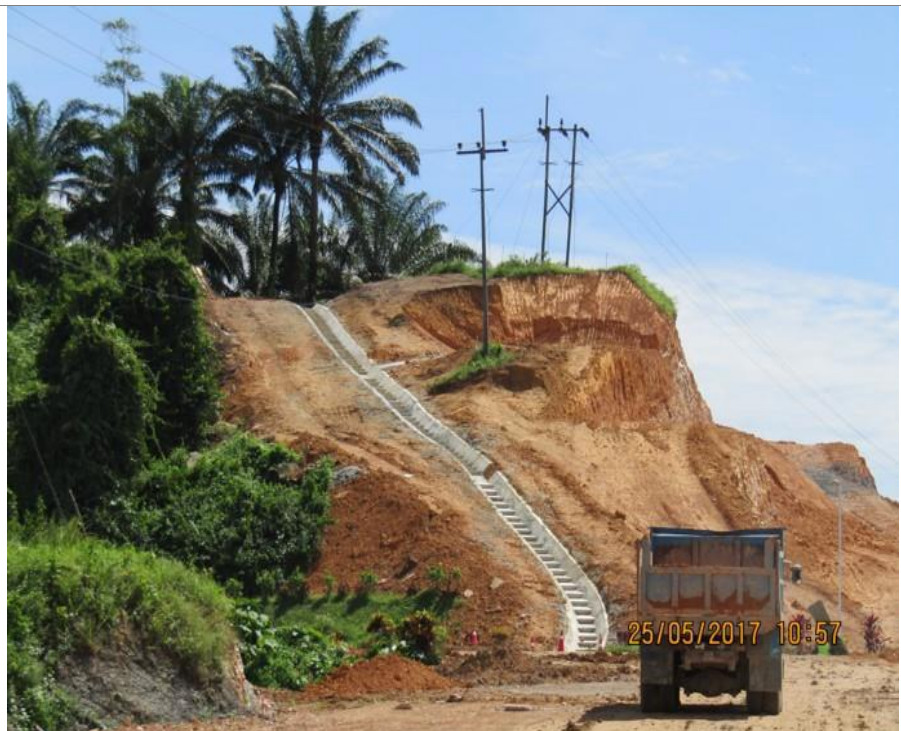
Chart 10 : Pan Borneo Works Package 5: Laying of interceptor drain (Spaoh Section)
