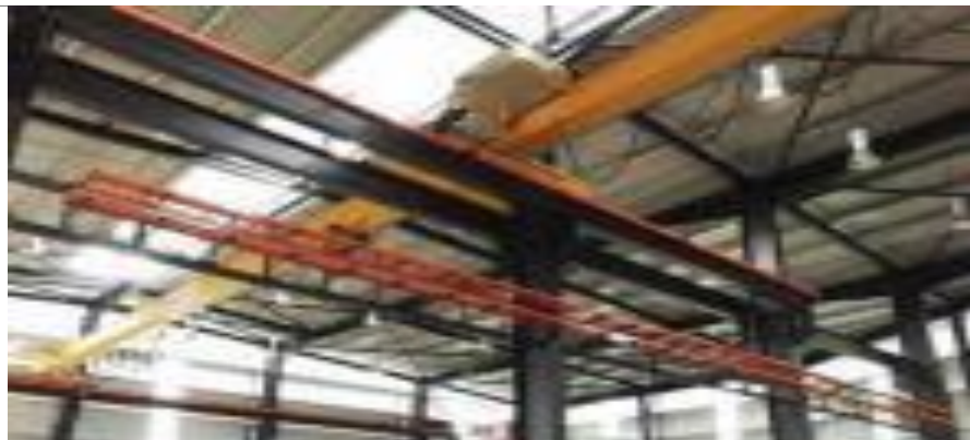
Chart 21 : Refit infrastructure works at the RMN Submarine Base, Sepangar Bay, Sabah
