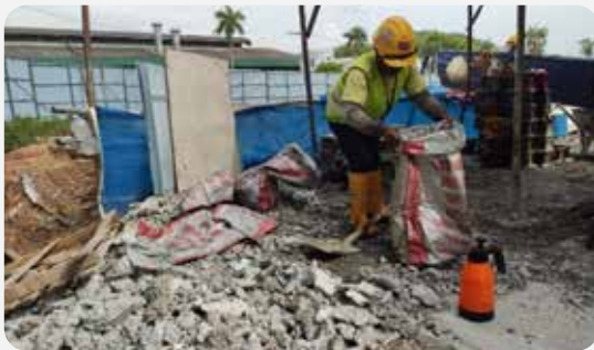
Used of hacked concrete as check dam
