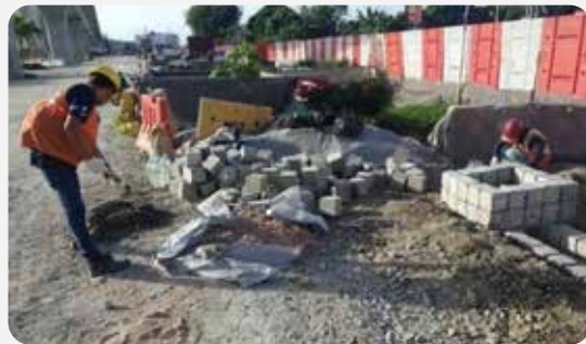
Used of test cube block for construction of temporary structure
