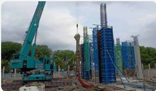
Usage of system formwork to reduce wastage of plywood from conventional formwork
