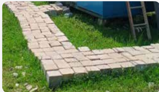
Usage of test cube block as walkway
