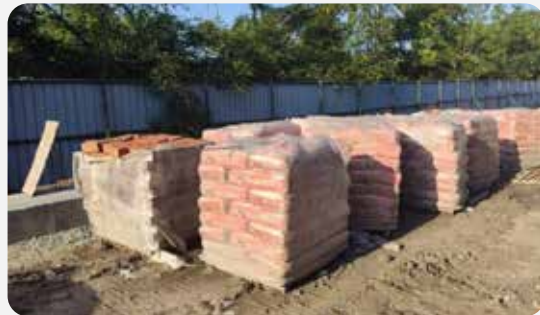
Proper protection of construction materials to prevent damaged/wastage
