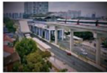
Facilities work for the Kelana Jaya Line LRT Extension Project
