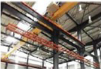
Malaysian Scorpene Refit Infrastructure Works at Sapangar Bay
