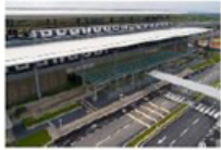
Elevated stations at Sg Buloh, Kg Baru Sg Buloh & Kota Damansara (MRT 1)
