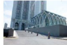
Alteration and Addition Works to Existing Kompleks Dayabumi
