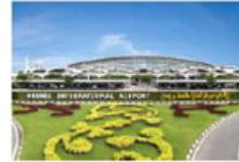
Modernization of Brunei International Airport Terminal
