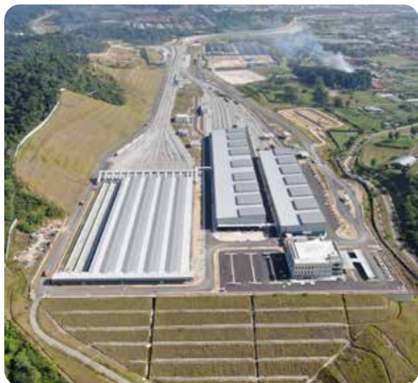
MRT Package DPT201, Serdang Maintenance Depot
