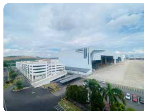
Completed SECA Project
